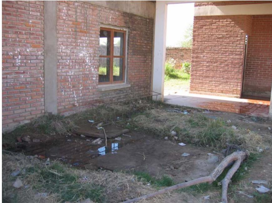
**Figure 3: Existing septic tank with standing water**
