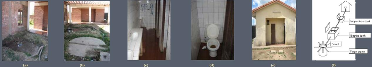
Figure 1: Existing conditions (a) Septic system (b) Pozo ciego (c) Flooding (d) Toilet (e) Toilet house (f) Existing system sketch
