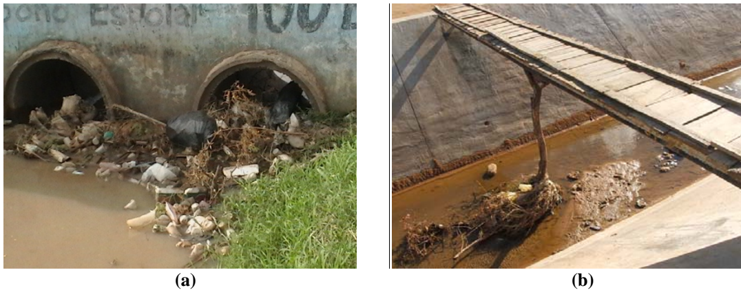
Figure 4.6: (a) - (b) Debris Accumulation in Drainage Structures: Photographs Taken in May of 2008 by C.C.E.
