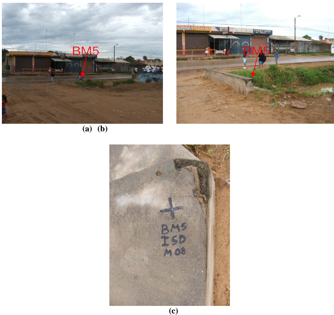
Figure B 11: (a) Location of BM 5 on the Nuevo Camino al Palmar Bridge to the Southwest of Avenida Fatima I (b) Close-up of BM 5 Location (c) Photograph of BM 5: Photographs Taken in May of 2008 by C.C.E.
