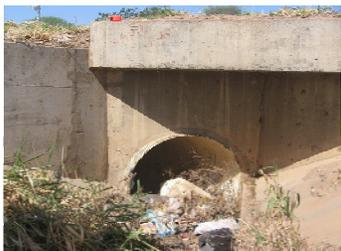
Figure 2: Culvert leading from existing canal to Doble Via. Regular cleaning of the existing and proposed canals is essential for proper functioning.
