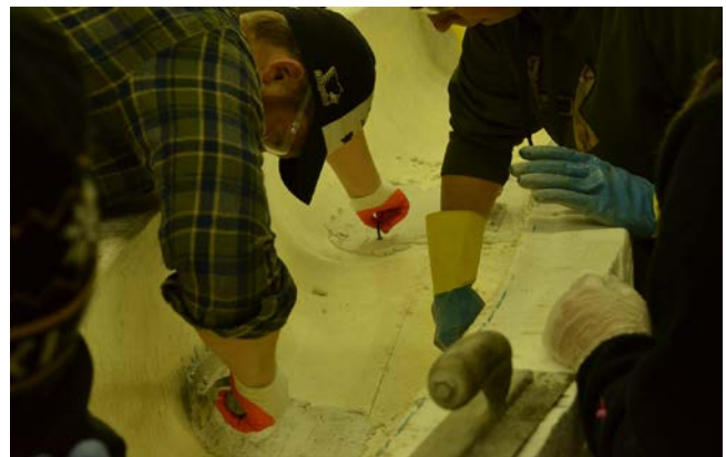
Figure 10: Concrete placement within Talvi Sielu
