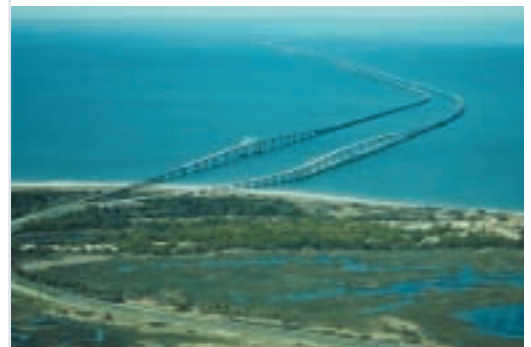
Chesapeake Bay Bridge Tunnel, Virginia
