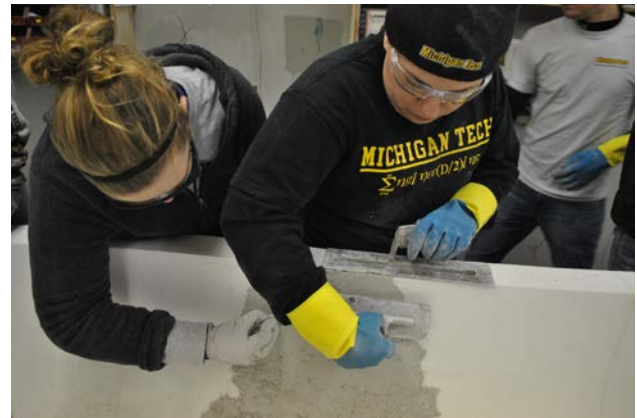
Figure 7: A troweler and QC member working together to ensure proper thickness.
