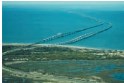
Chesapeake Bay Bridge Tunnel, Virginia
