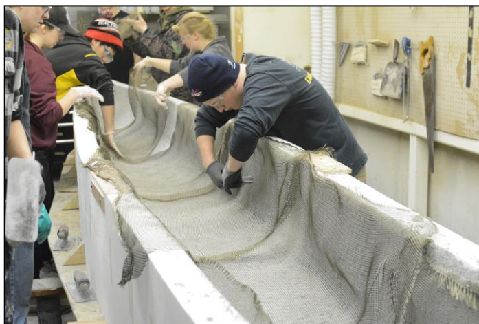
Figure 6. QC/QA monitors applying the primary reinforcement
