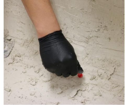
Figure 6: Verifying Concrete Depth
