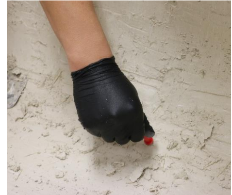
Figure 6: Verifying Concrete Depth
