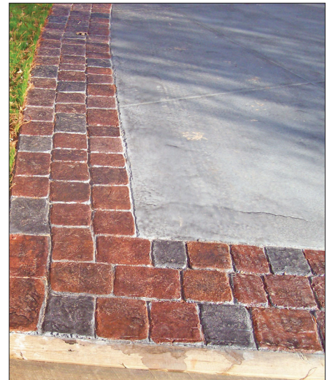
Close-up of stamped concrete walkway as shown above (Photo Courtesy of Decocrete)
