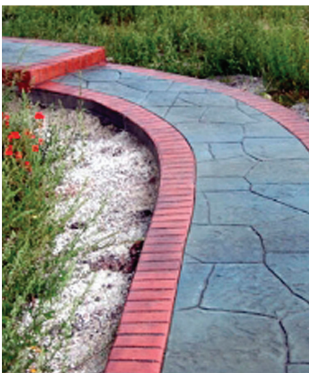
Stamped walkway colored with Direct Colors Pigment (Photo Courtesy of Mark Douglass)
