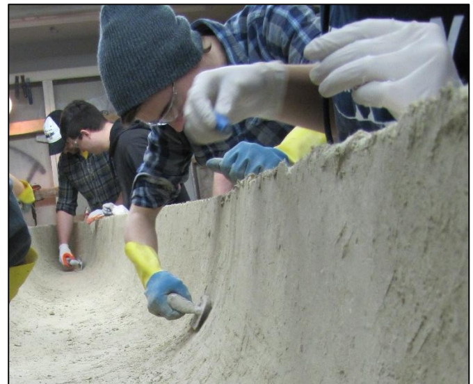
Figure 11: Concrete Placement
