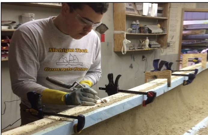
Figure 13: Troweled Gunwale Caps
