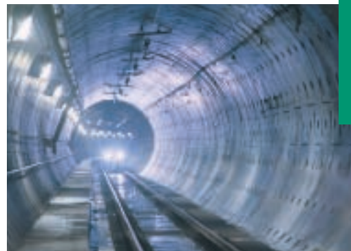
Light rail tunnel leading to the Minneapolis-St. Paul International Airport
