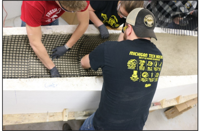
Figure 12. Reinforcement Placement
