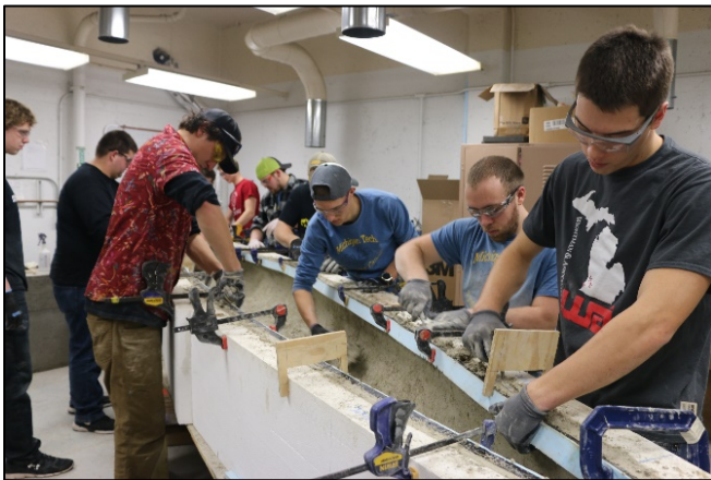
Figure 13. Gunwale Cap Construction
