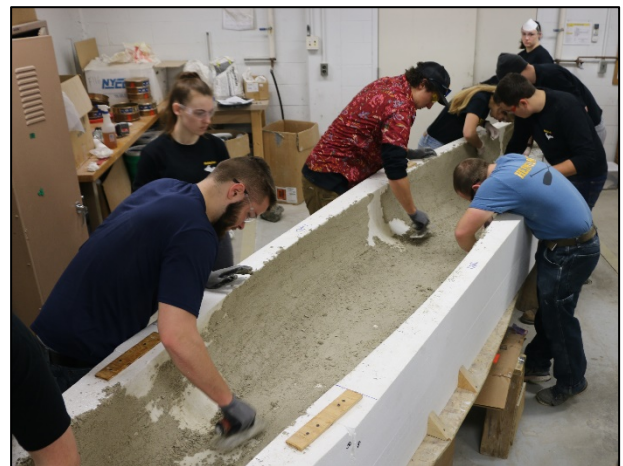
Figure 11. Application of the First Layer of Concrete
